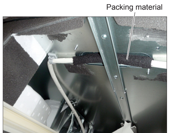
<After replacing the motor>
