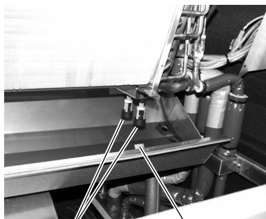
Float switch X2 Drain pan fixation point
