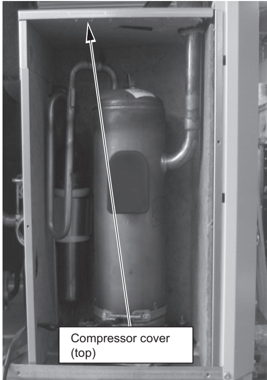
4. Remove the compressor cover (top).
