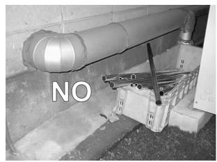
Store the pipes to be used indoors. (Warehouse at site or owner's warehouse) If they are left outdoors, dust, dirt, or moisture may infiltrate and contaminate the pipe.
