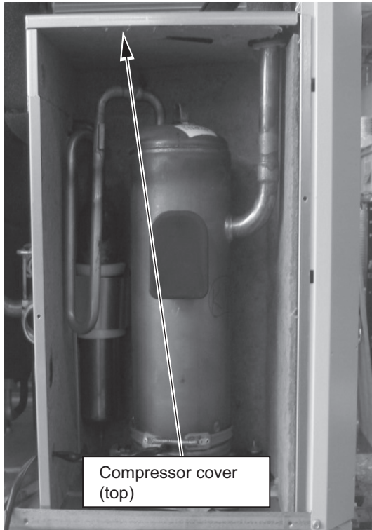
4. Remove the compressor cover (top).
