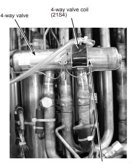
4-way valve coil fixing screw
