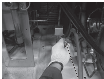
Refrigerant charge port (CJ3)
