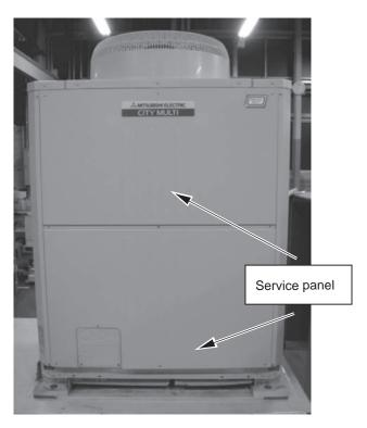
1. Remove both the top and bottom service panels (front panels).
