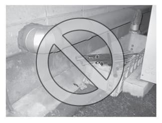
Store the piping materials indoors until they are ready to be installed (e.g., storage room on site or at the installer's premise). If left outdoors, dust, dirt, or moisture may infiltrate and contaminate the pipe, resulting in malfunctions.
