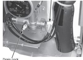
Drain cock (Pump valve side)
