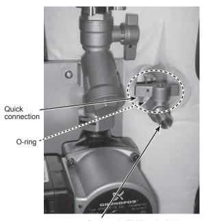
Drain cock (DHW tank side)
