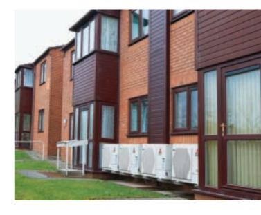
One 5kW Ecodan unit was installed for every two flats, providing heat via a radiator circuit fitted with independent lockable heating stats and thermostatic radiator valves, further helping to save energy costs.
