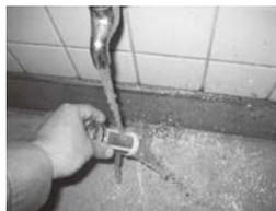
5. After the power to the HBC controller is turned on and the system starts up, set DIPSW4-6 and DIPSW4-7 to ON. Turn off the power to the HBC controller again, and clean the other strainer furthest from the water supply. (After the cleaning, set DIPSW4-6 and DIPSW4-7 to OFF.)
