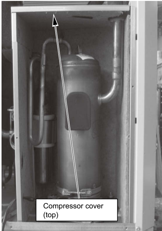
4. Remove the compressor cover (top).
