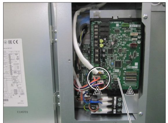
Control circuit board
