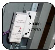
The Filter Indicator pcb is now accessible to change the jumper position.
