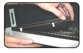
The grille filter can now be unclipped from the grille and brushed and vacuum cleaned.
