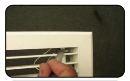
Then push the grille core sideways against the spring loaded pins on one side and the grille core with filter now comes clear of its frame.
