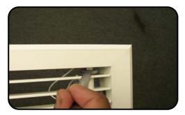
Towards the rear of the recessed grille (nearest the doorway), and at each end of the grille, there are two conical bolts that prevent the grille being removed without the use of tools.
