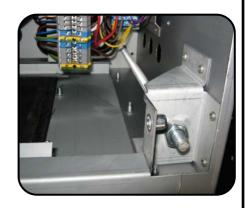
Four of the threaded rods (the two at each end of the unit) enter the casing from above and are attached to fixing brackets near the bottom of the unit (see photo above – looking up into the air curtain). The two centre threaded rods (on PHV1500 and PHV2000 units) are attached to the top face of the casing.
