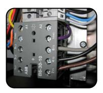
Wiring to the air curtain should be carried out in accordance with the wiring diagram on Page 12 and IEE Regulations. The figure below shows the completed wiring for a 3 phase electrical supply if the defrost electric heaters are required.
