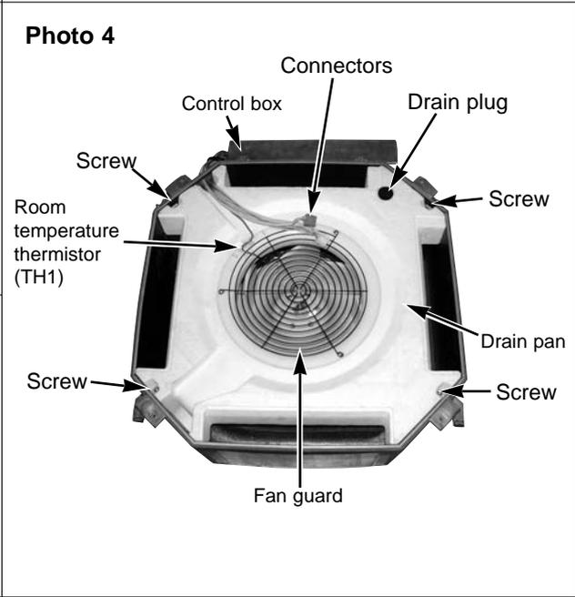
**6. Removing the drain pan**
